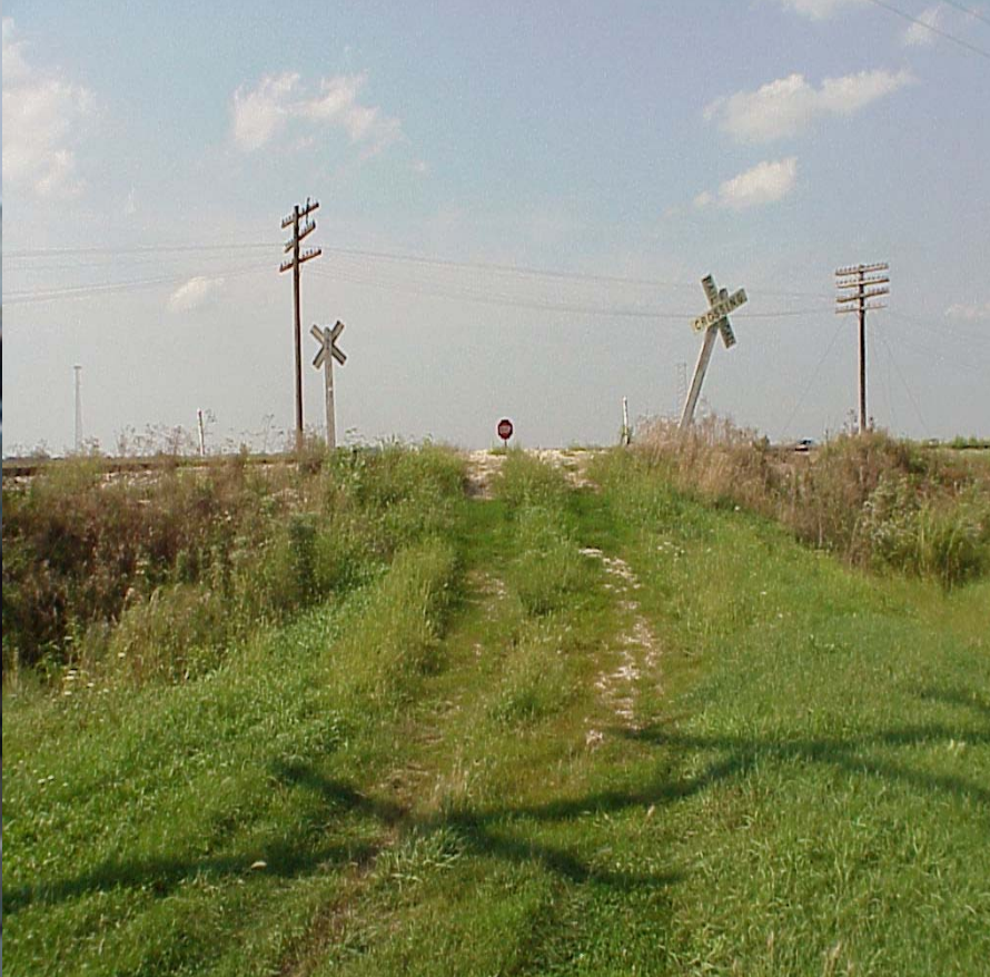
Field Crossing w/o Active Warning Devices
